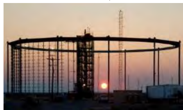
Infrastructure in place with state-of-the-art equipment
